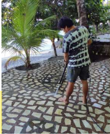
Removed algae using high pressure
