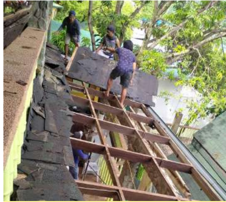
Repaired and replaced damaged roof
