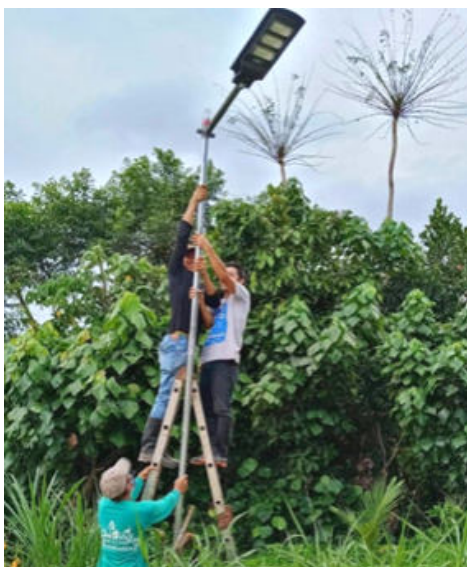
Installation of Additional Solar Street Lights
