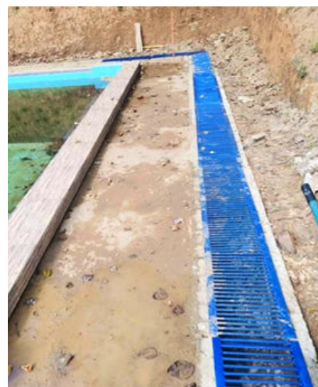
Water Canal, Fabricating Grill Cover for Swimming Pool
