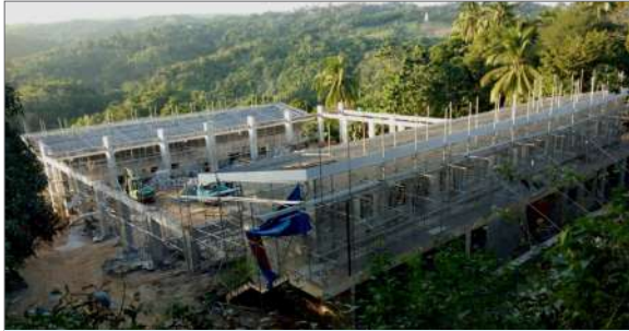
Multi Purpose Building Construction (MPB)
